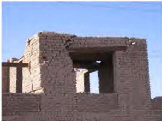
(b) Simple Masonry (Vulnerability class B)
